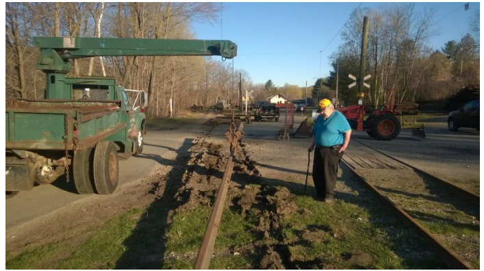
John Greene inspects track repairs in 2007
