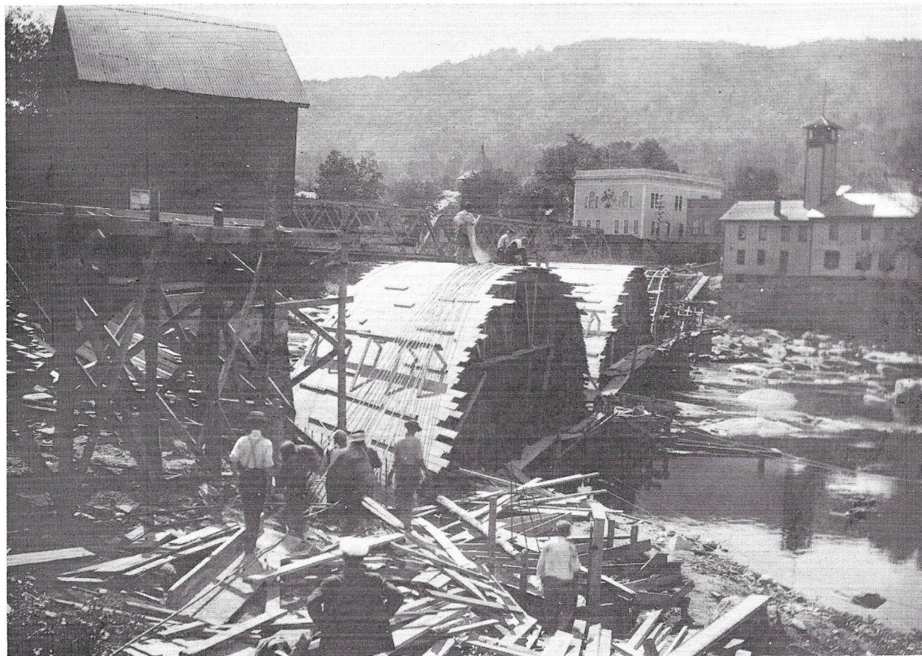
AUGUST 19, 1908—"The bridge contractor is now constructing the falsework necessary to support the concrete arches," the Shelburne Falls Messenger reported for that date. Photos showing bridge construction were loaned by courtesy of Mrs. Madeline Reed Scranton, daughter of Frank L. Reed, street railway superintendent 1907-1914.
