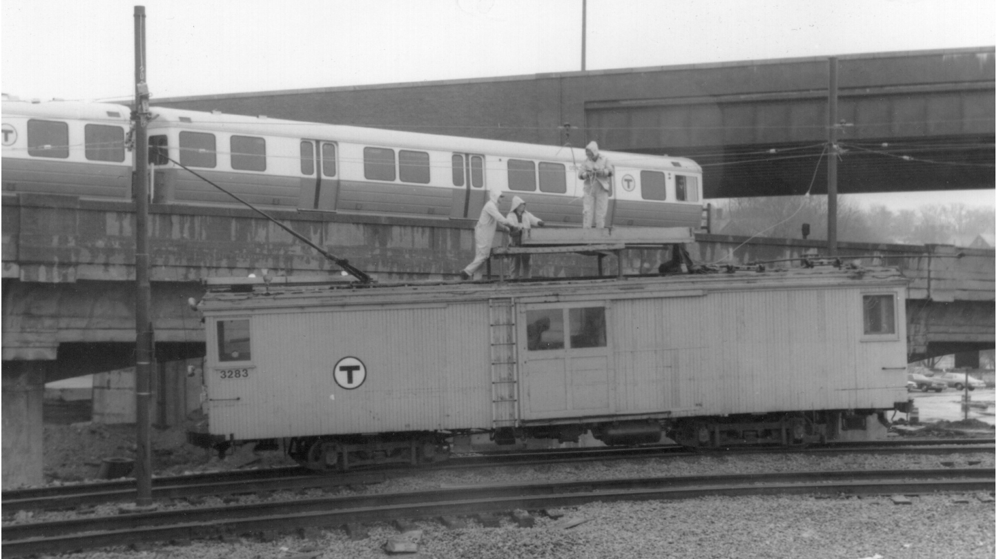
MBTA Line Car 3283 at work in Forest Hills, Mass. in 1984. Note that the work platform has been raised to allow access to the overhead wire. Photo by Norton D. Clark, Kevin Farrell Collection
