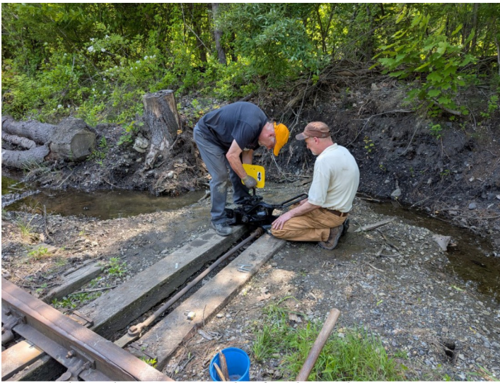
Nash and Martin put the final touches on a "new" switch stand for Turn Out 4.
